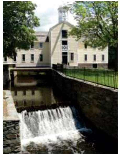
Samuel Slater's first mill, built in 1793, still stands in Pawtucket, Rhode Island
